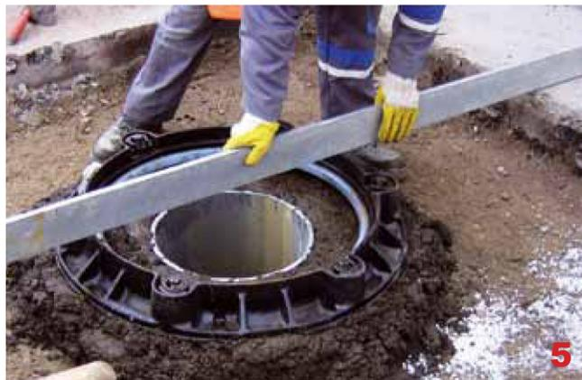
**5** Lay the frame directly on the sealing product.
