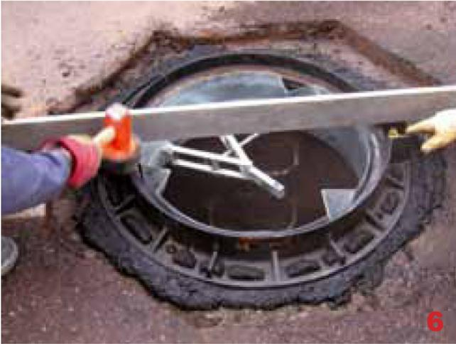
**7** Check that the frame openings have been completely filled.
