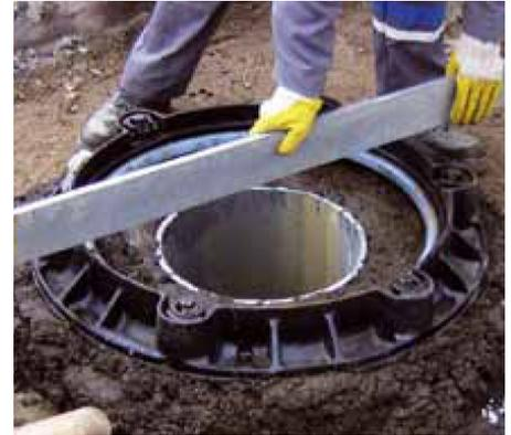
**1** Check the diameter of the manhole opening or groove that the frame is to be fitted on.
