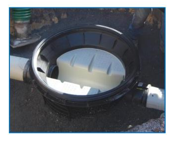
For all sockets horizontal angles of  $\pm$  3.75° or gradient changes up to 6.5% are possible. Direction and gradient changes at the same time will reduce the indicated maximum values accordingly.
