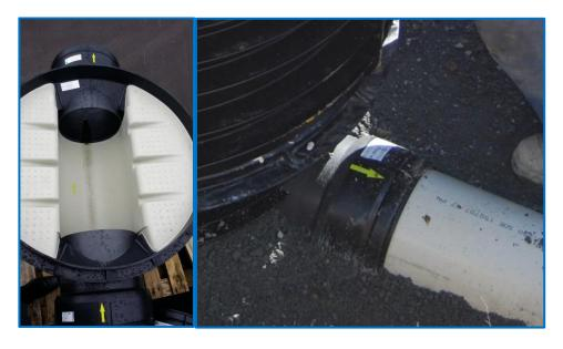
The Base should be checked with a spirit level to ensure that it is sitting level on the bedding.
