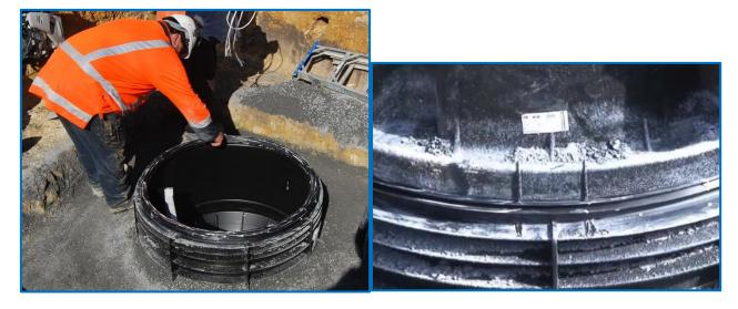
Align all manhole elements according vertical marks on the outside of the Riser and Cone elements to ensure the alignment of the ladder.
