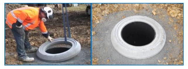
Below the LDR the bedding must be planar and free of point loads (consider using grit, sand or concrete dust). For class D applications, this should be prepared according to the design requirements for the road base course.
